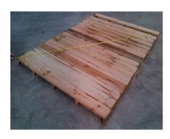
Step 3: Nail plastic weather strip to edge of floor on all four sides, with 30mm clouts, (approx 5 nails per side) ensuring top edge is flush with top of floor. This isn't required if shed is on a concrete base.
