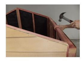
Step 10: Using 30mm clouts nail top cedar boards to stiffeners (2-3 nails per board). Predrill holes to stop boards from splitting.
