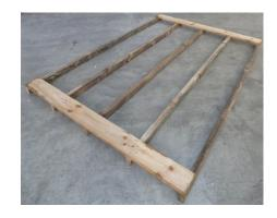
Step 2: Lay out remaining floor boards. Measure diagonals to ensure measurements are equal (i.e. floor is square). Rip down last floor board to suit gap, and nail off floor with 50mm flooring nails (12 nails per board).
