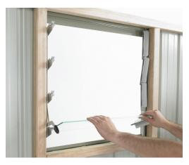
**Step 6:** From the inside of the shed, slide Louvre Glass into Louvre Units attached to the Window Frame. Bend up tabs to keep Glass in position.
