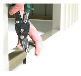
**Step3:** Measure and cut Doorstep Flashing (106) to fit in between Door Jambs. Position the Doorstep Flashing in between the Door Jambs at bottom of doorway, nail through top of flashing using three 30mm Clouts. Repeat with the Overdoor Flashing (105).
