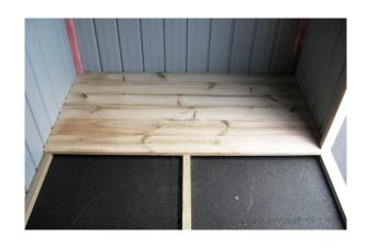
Step 4: Nail in each Floor Board, two 50mm nails in each end and two into Joist. Measure and cut Floor Flashing (110) to fit in between Door Jamb Flashings and nail in place using 50mm Clouts.
