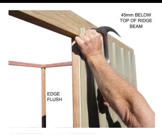
Step 2: Back Wall: Position the first Wall Sheet with the LIP on the right hand side. Ensuring the LIP is flush with the side of the corner Stud and the top of the Wall Sheet is flush with the top of the Top Plate, tack in place. Position the next Wall Sheet with the LIP on the right hand side. Overlap as shown in *fig 1*. Ensuring Wall Sheet is flush with top of Top Plate, tack in place.
