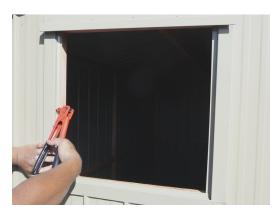
Step 6: From the outside of the shed, place glass in Window Frame. Attach a Glazing Bead (G100) with three rivets to each side of the Window Frame to hold glass in place. Predrilling Glazing Beads is recommended.
