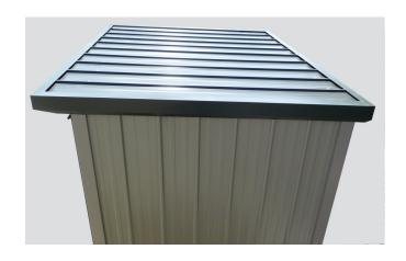
Step 2: Centralise Barge Flashing on end and rivet in place, one rivet into every second Rib. Fit two rivets through top of Barge into Rib. Repeat with other Barge Flashing. Check Spoutings are straight, then rivet to Roof one rivet every second Rib.
