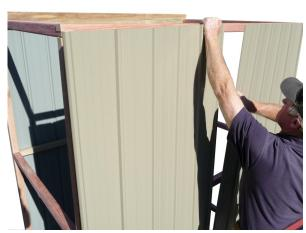
Step 3: End Walls: Position wall sheet with the LIP flush with the side of the stud and the top of the Wall Sheet is flush with the top of the Top Plate, tack in place. Tack in remaining 1/2 Wall Sheet. Repeat with the other end. If fitting a window, nail in Window Studs and Nog now. Refer to Window instructions.
